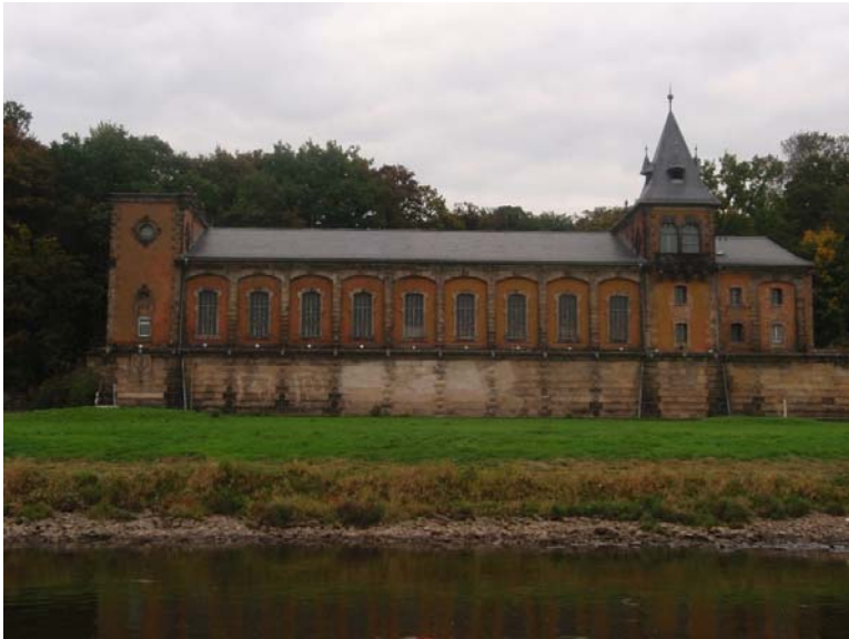
Water supply works on the Elbe River in Dresden Germany
