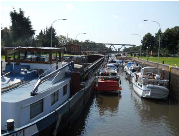
Commercial and recreational navigation together in a lock
