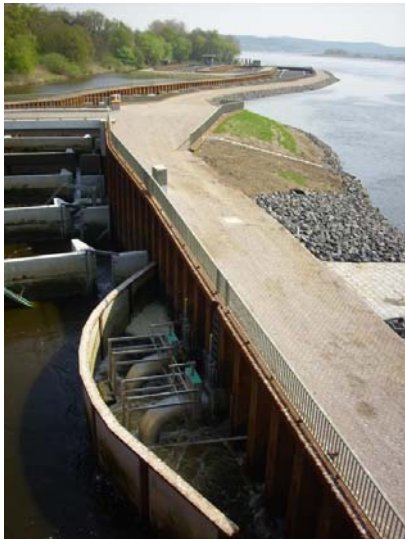
Fish way in Geesthacht, Elbe River, Germany
